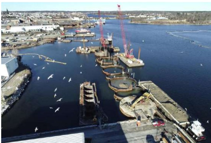
Figure 4-4: left: CAD-cell in Port of New Bedford, Massachusetts
